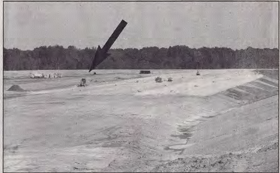
The rail yard bed is being constructed.
