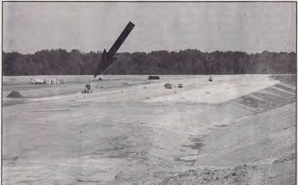
The rail yard bed is being constructed.
