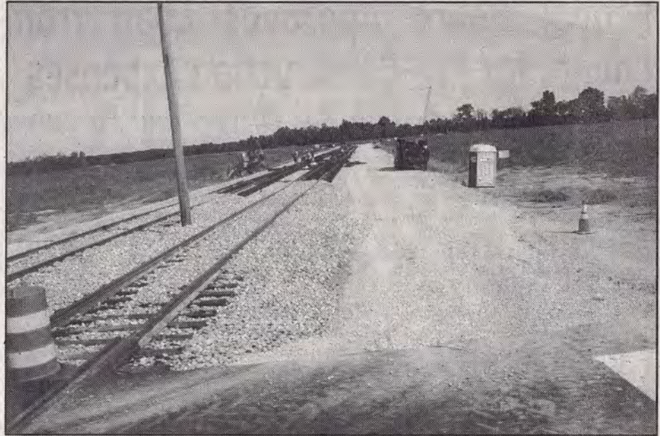
New railroad track is being constructed crossing Highway 57 near Rossville.
